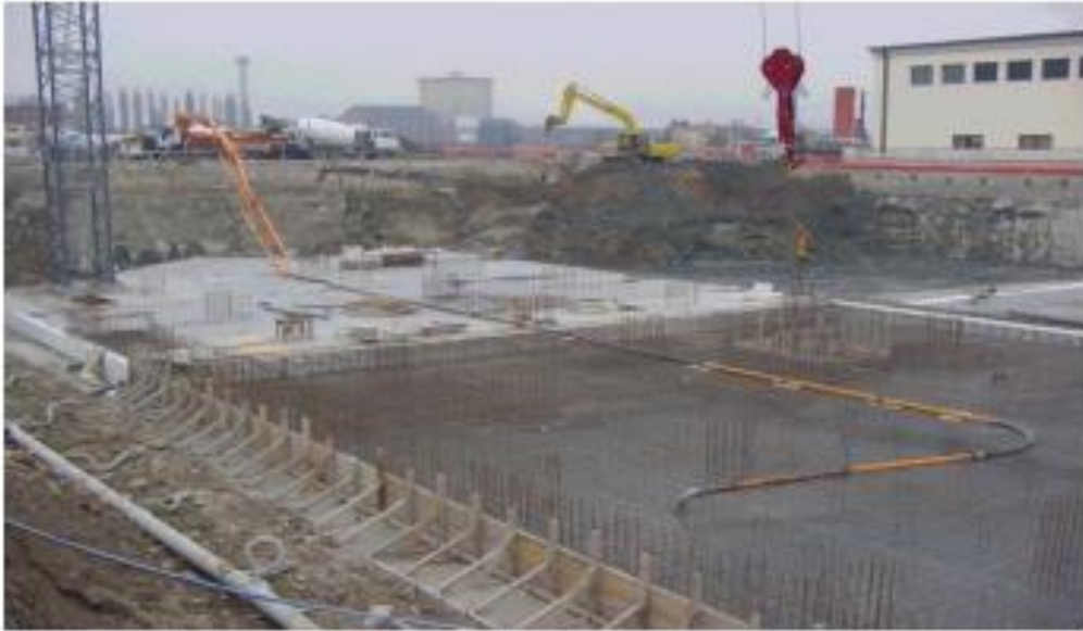
Figure 11.1: Casting an SCC slab. Commercial centre, Ferrara, Italy.
