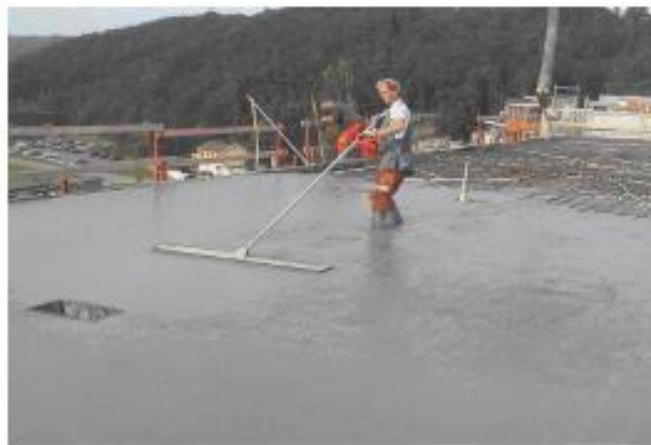
Figure 11.1 Levelling SCC with a skip float
