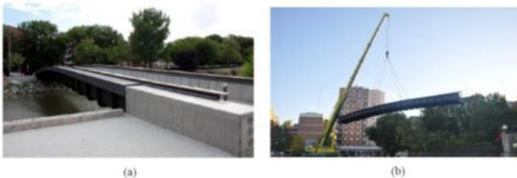
(a) View of the Almuñecar footbridge; (b) Installation of the FRP girder.
