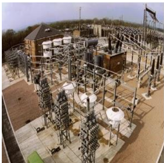
SVCs (Static VAr Compensators)
