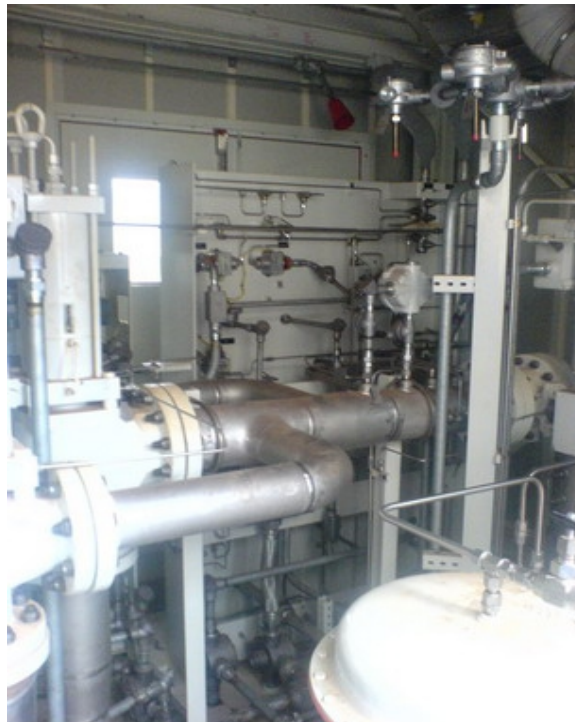
ΕΙΚΟΝΑ 18: 3 αγωγοί (PRIMARY-SECONDARY-TRANSFER)
