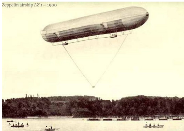
Graf von Zeppelin's LZ1, the world's first successful rigid airship
